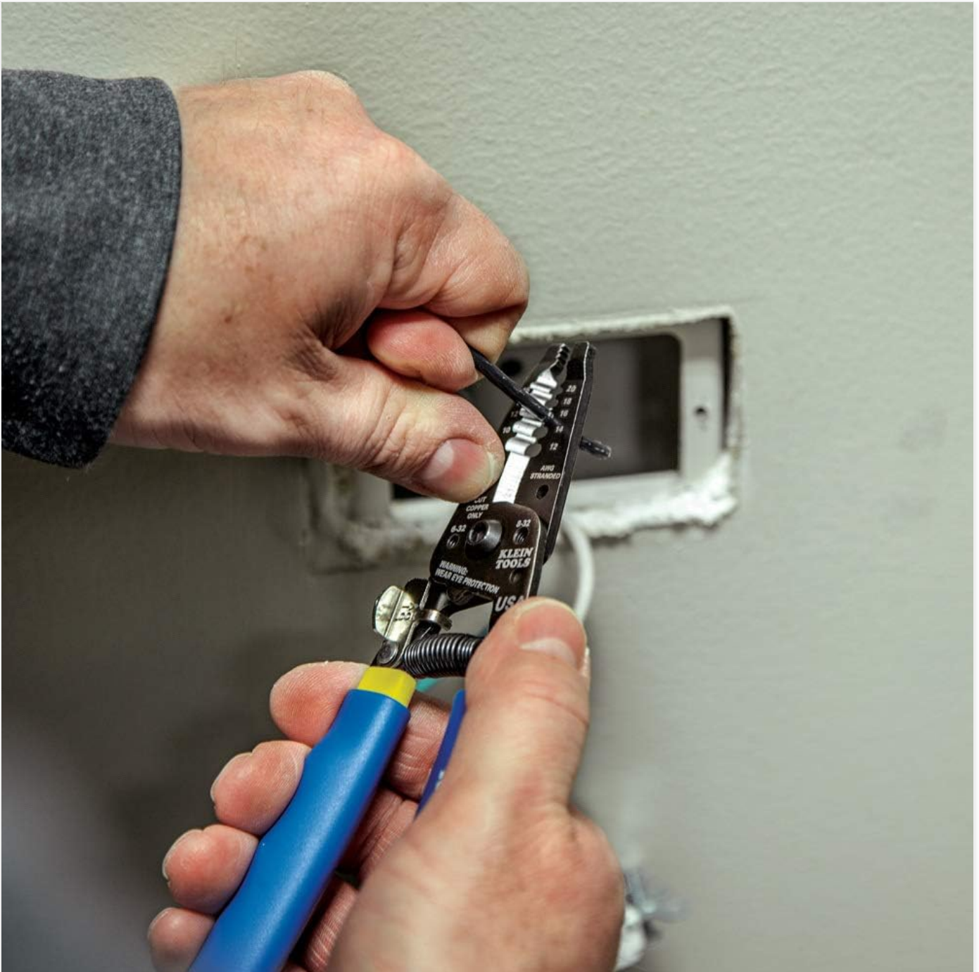
Figure 3: Proper technique for stripping wire insulation.
