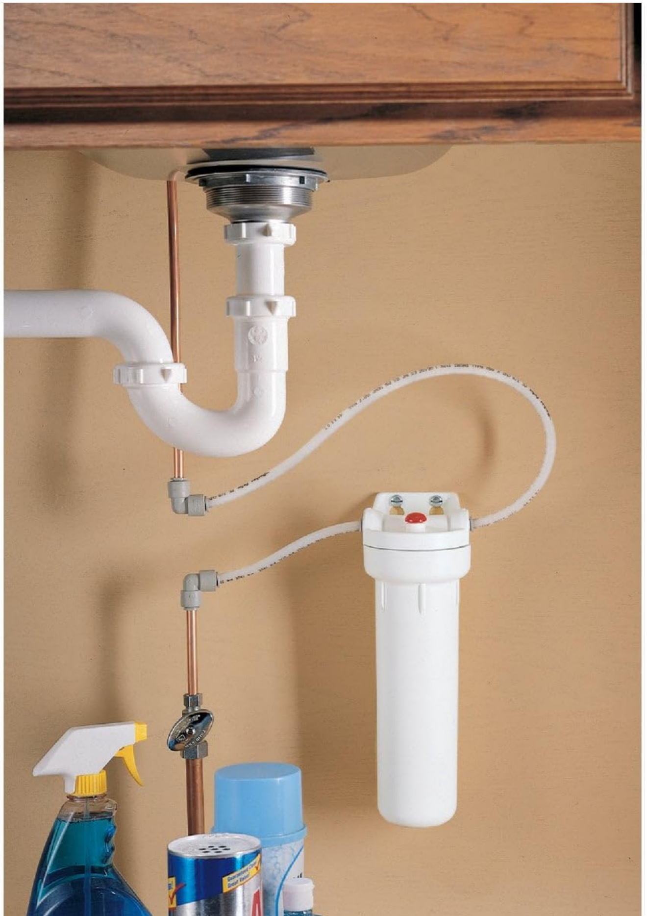
Figure 5.1: Example of the Culligan US-600A system installed under a sink, showing connections to the cold water line.
