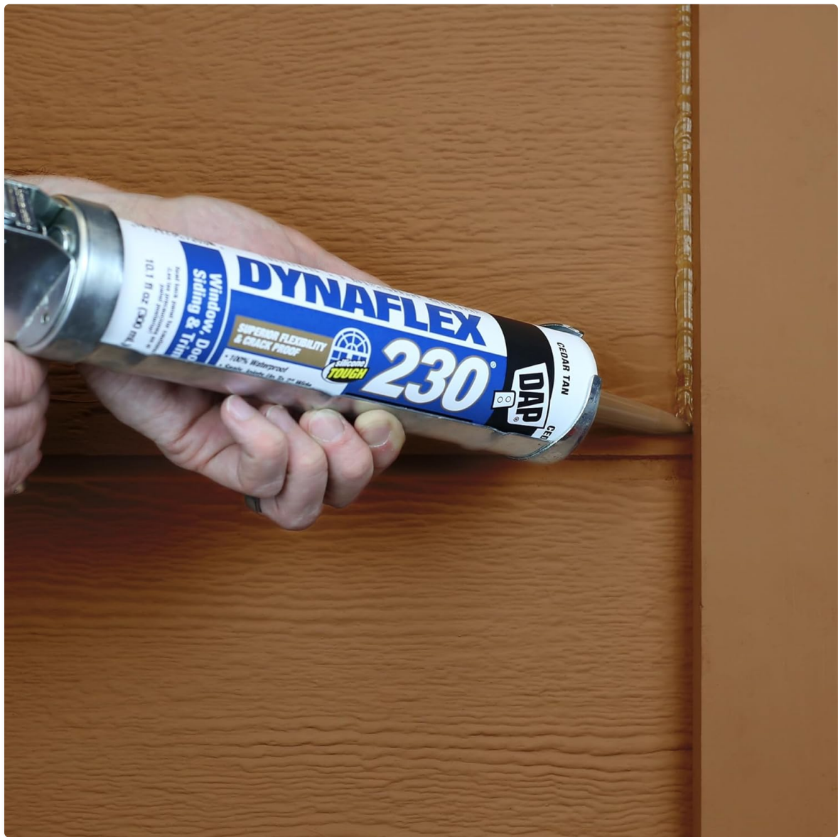
Image 3: A hand demonstrating the application of DAP Dynaflex 230 sealant using a caulk gun along a wooden seam.
