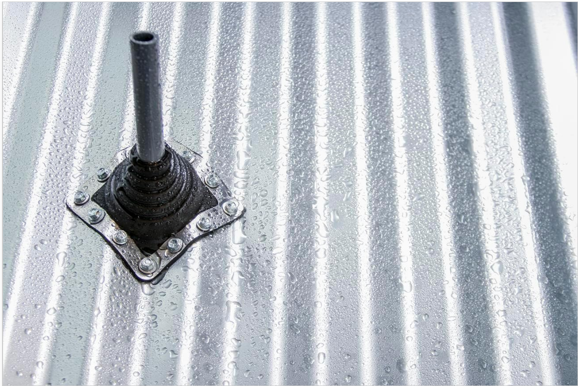
Image: An Oatey Master Flash Roof Flashing securely installed on a corrugated metal roof, fastened with screws around its perimeter.
