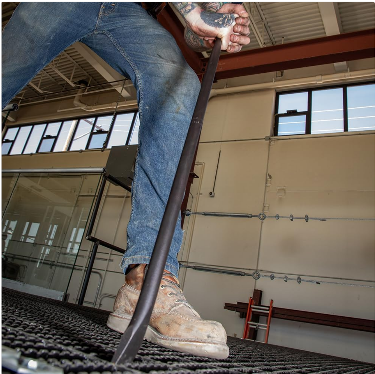
Figure 5: A close-up view of a worker using the connecting bar to gain leverage. The angled chisel end is positioned for maximum mechanical advantage.
