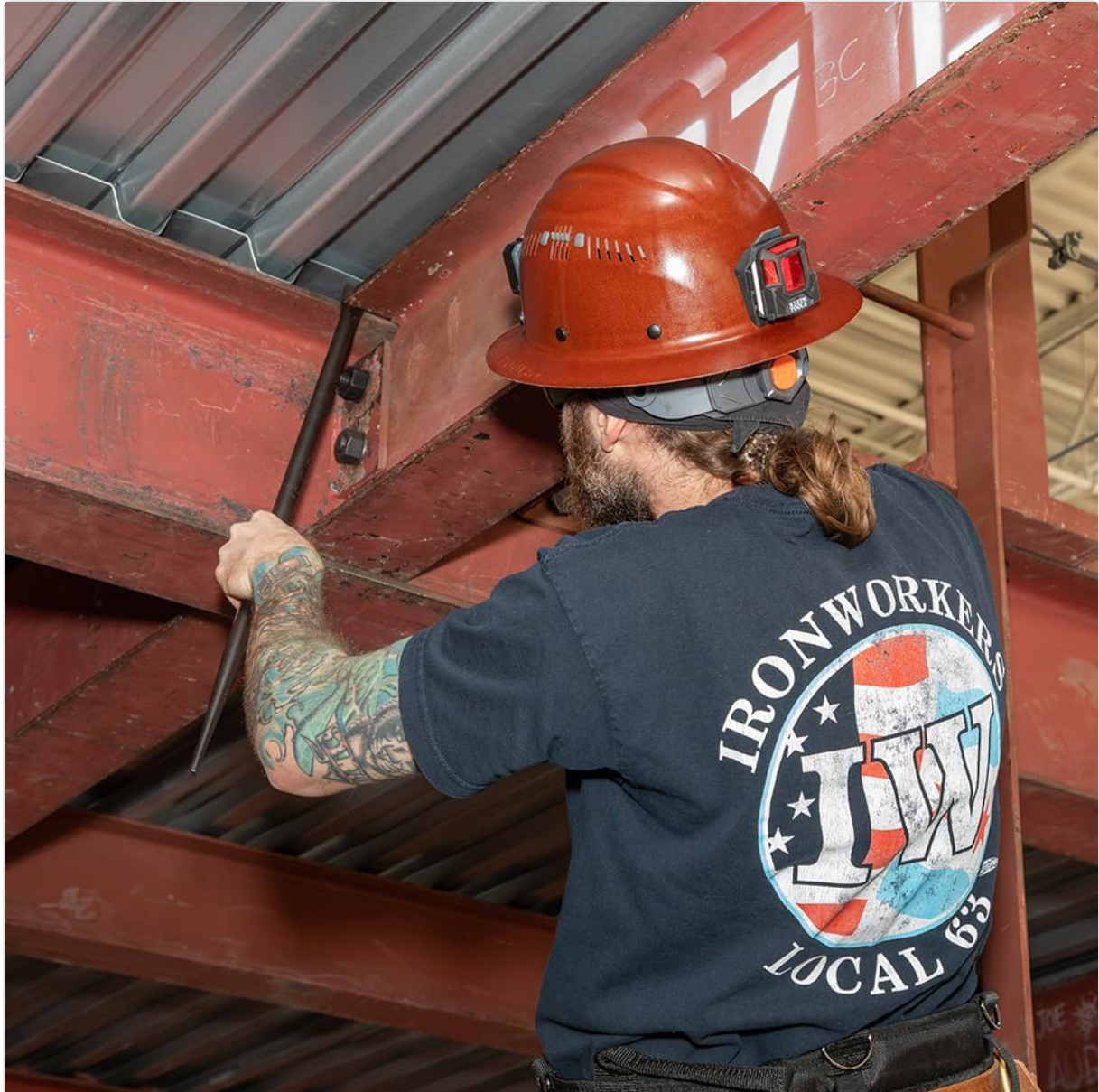
Figure 3: A worker using the Klein Tools connecting bar to align bolt holes in a steel beam. The tapered end of the bar is inserted into the holes to facilitate precise positioning.
