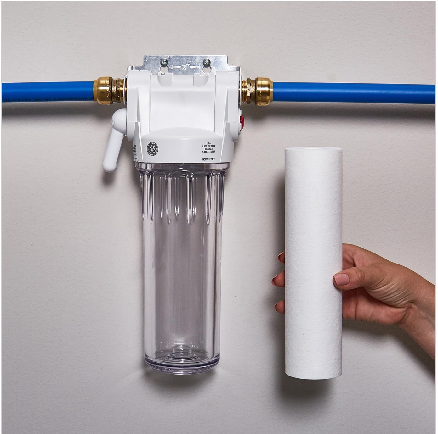
Image 5: A new filter cartridge ready for replacement next to the existing filter housing.
