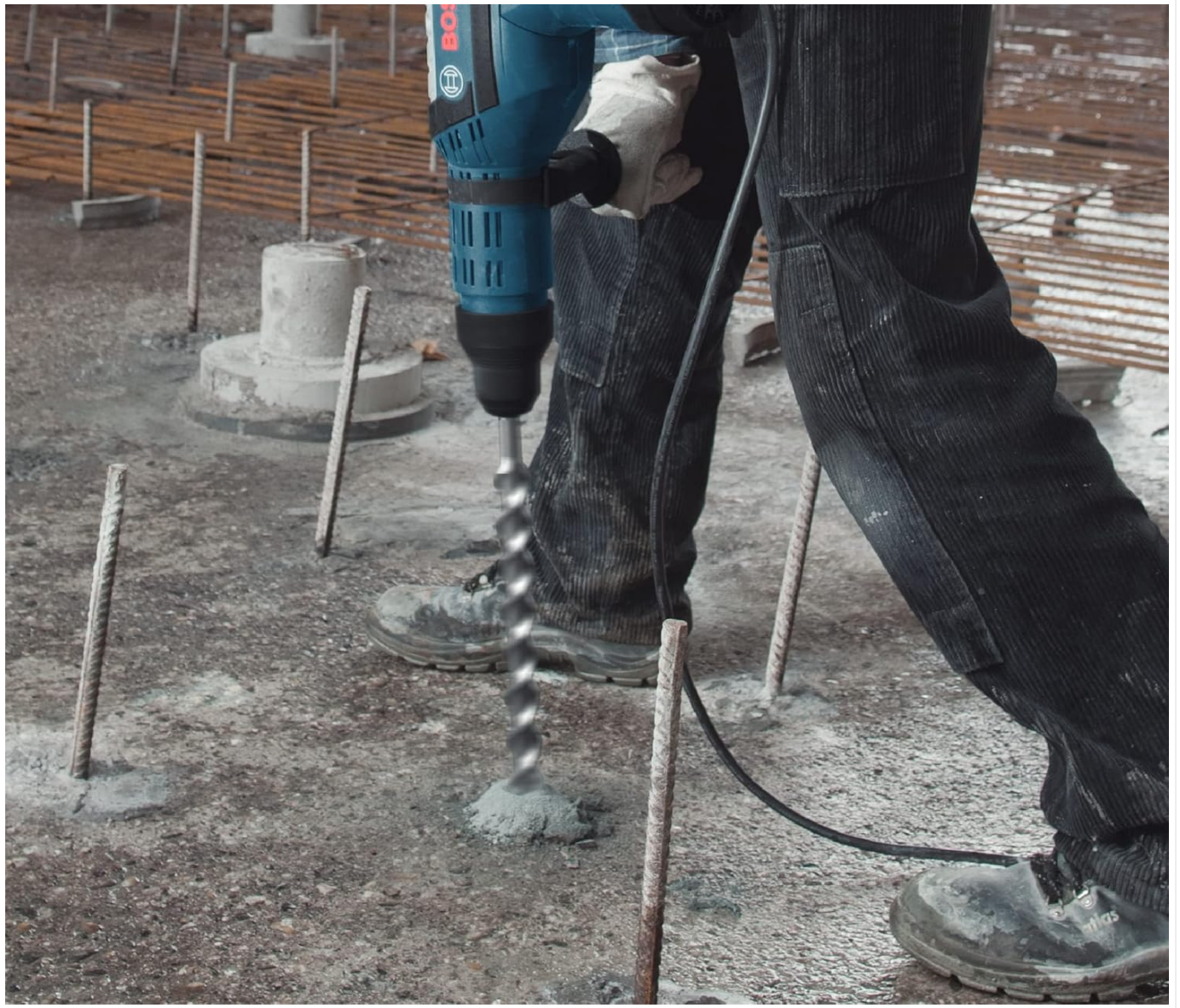
Image: A close-up view of the Bosch SDS-max Speed-X bit actively drilling into a concrete surface, showing dust being expelled.
