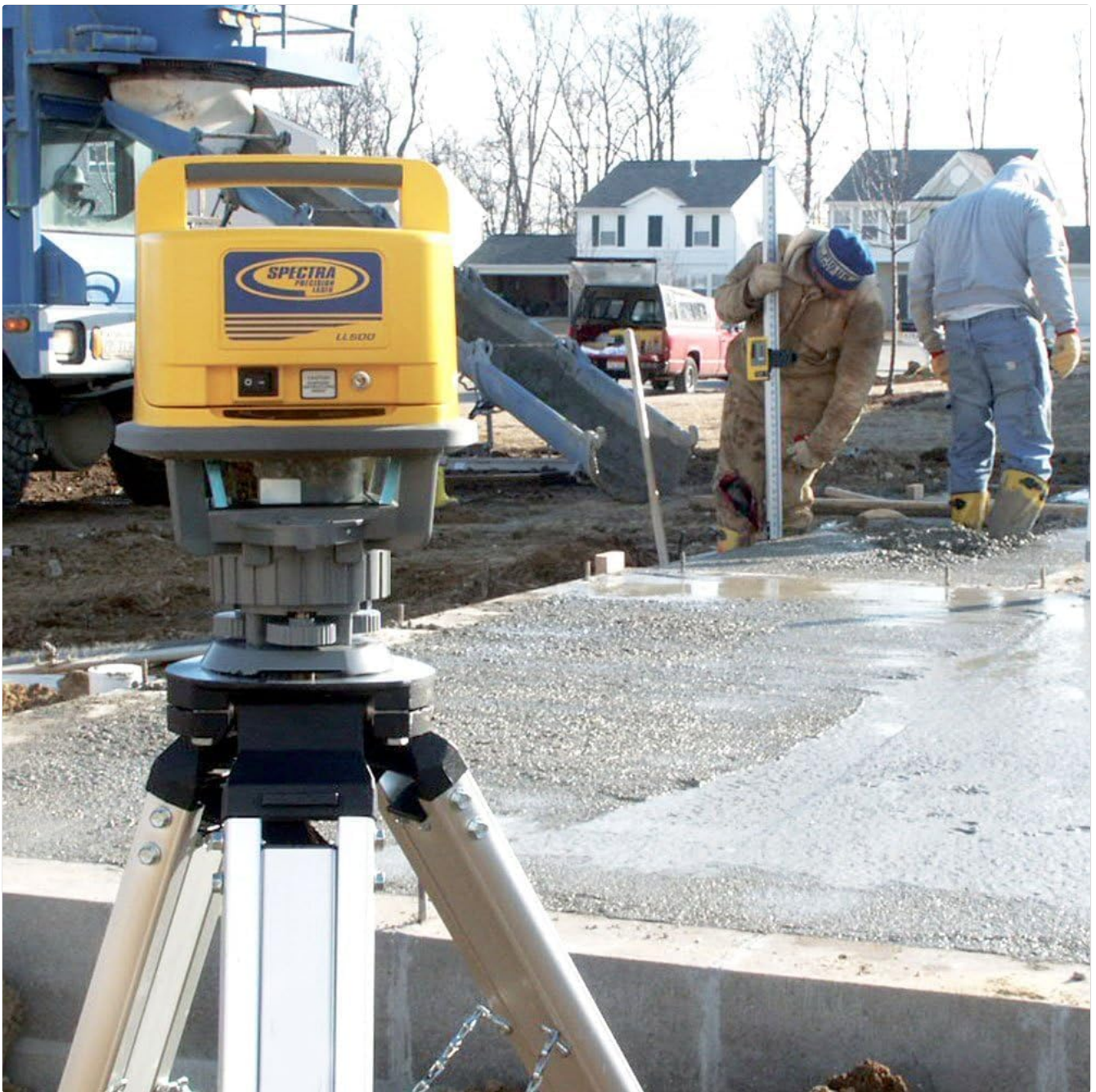
Figure 6: LL500 Laser Level assisting with concrete formwork.
