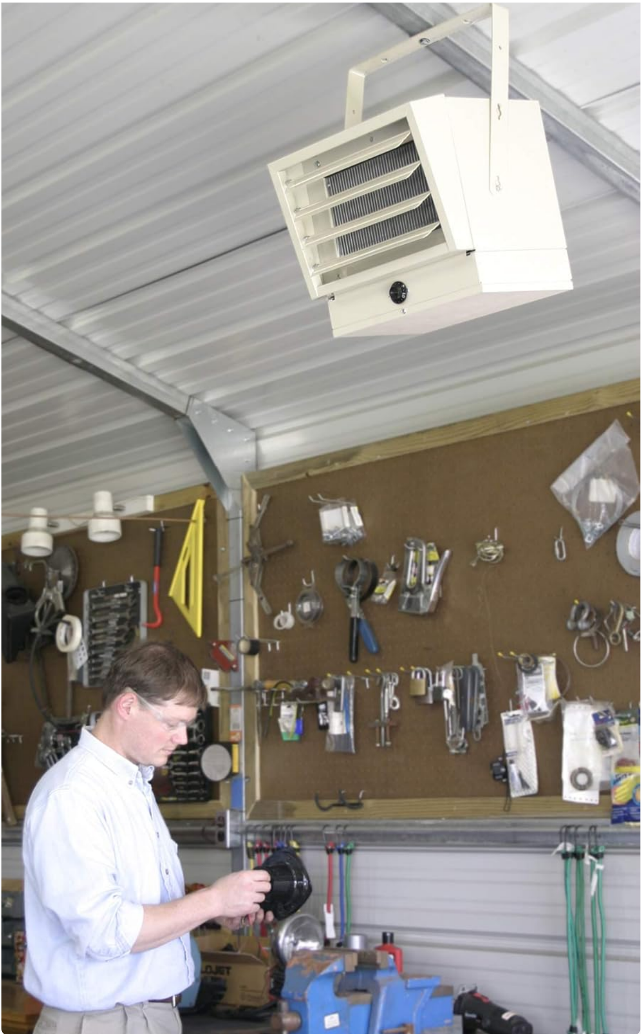
Figure 3: Fahrenheat FUH54 Electric Heater mounted on a ceiling, providing warmth to a garage space.
