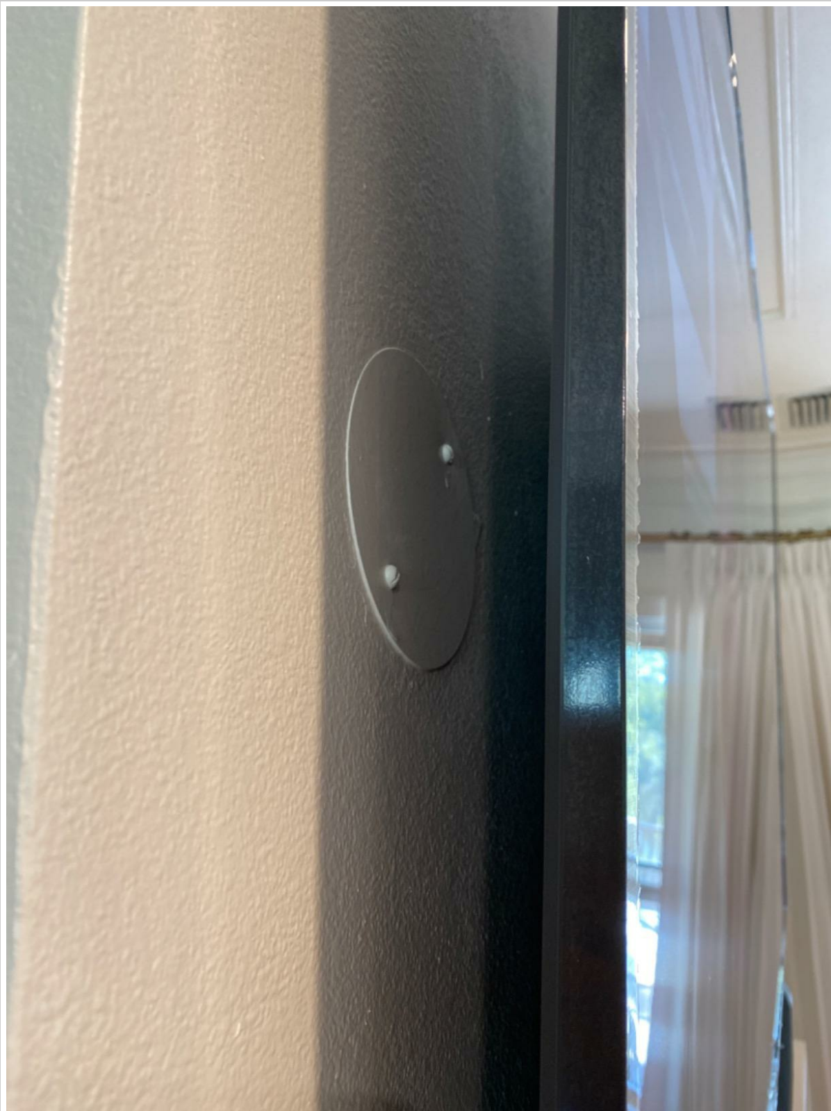
Image 5.1: Example of the outlet concealer painted to blend with the wall color.
