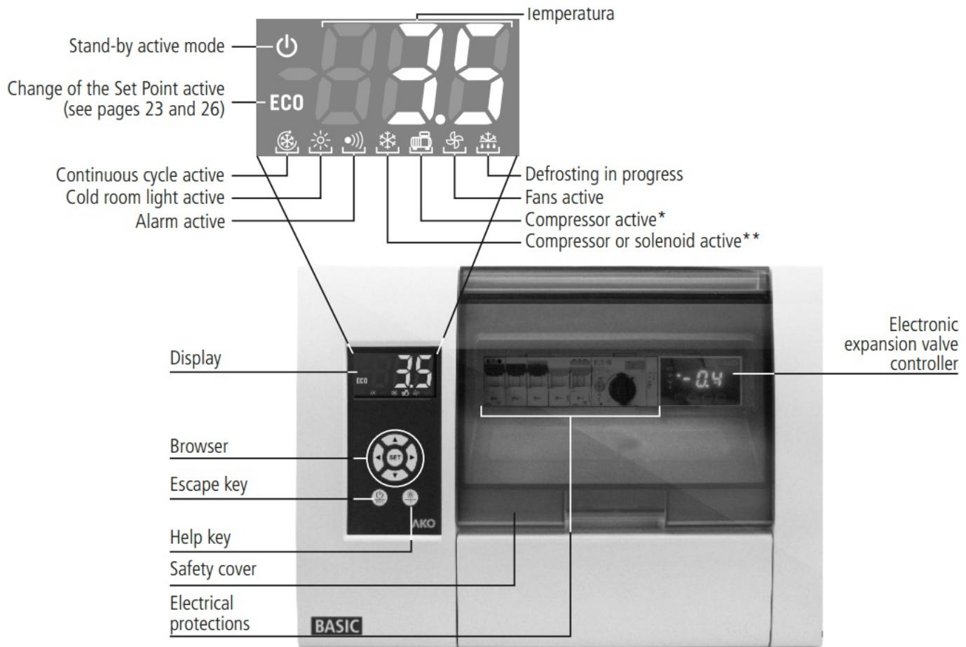
If pump down is active, it indicates the operation of the compressor.
