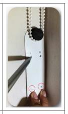
3. Now drill into the markings to create holes for the screws Now screw the bracket onto the wall.
