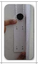
2. Now use a pencil to mark the hol es for the screws. If you're installing the motor on the left of the the wind ow use the "L" marking and "R" marking to install on the right
