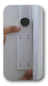
2. Now use a pencil to mark the holes for the screws. If you're installing the motor on the left of the the window use the "L" marking and "R" marking to install on the right
