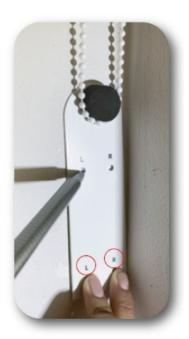
3. Now drill into the markings to create holes for the screws Now screw the bracket onto the wall.
