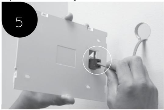
Pull in the cable from the hole and connect it to the RJ12 socket. (Part number #657258)
