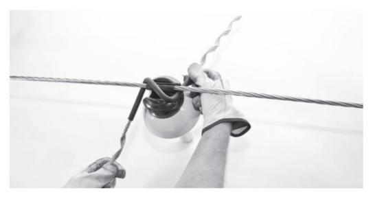
5. Bend one leg of the Longspan Tie around the neck of the insulator. Ensure the Tie is firmly seated under the insulator ear.
