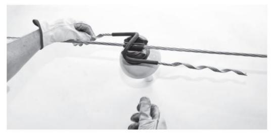
4. Rotate the Longspan Tie counter-clock-wise. Ensure both legs go under the conductor. Rotate the Longspan Tie until the legs seat themselves.
