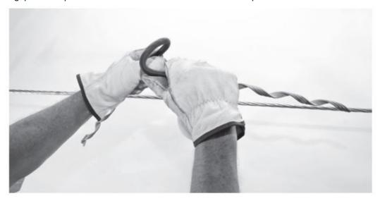
3. Install the Longspan Tie over the center of the insulator so that both legs are parallel to the conductor.
