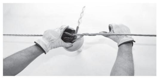
6. Continue wrapping the Longspan Tie legs until it is completely wrapped.
