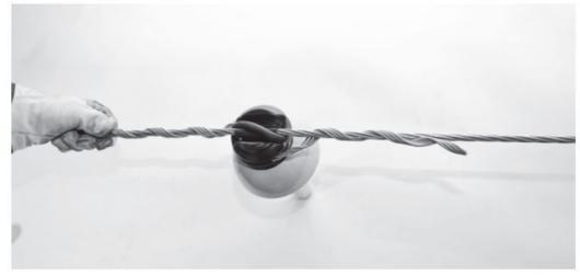
7. Snap the end of each leg into place. Ensure the Longspan Tie end fully snaps into place. This may require more pressure than the pressure to wrap.
