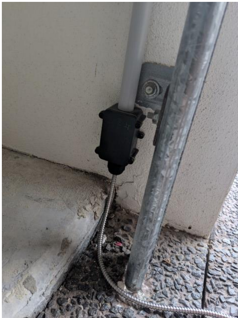
Garage Door Sensor – Installation Example – on the ground
