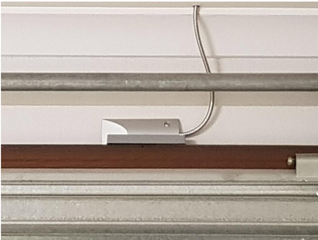
Garage Door Sensor – Installation Example – on the ground
