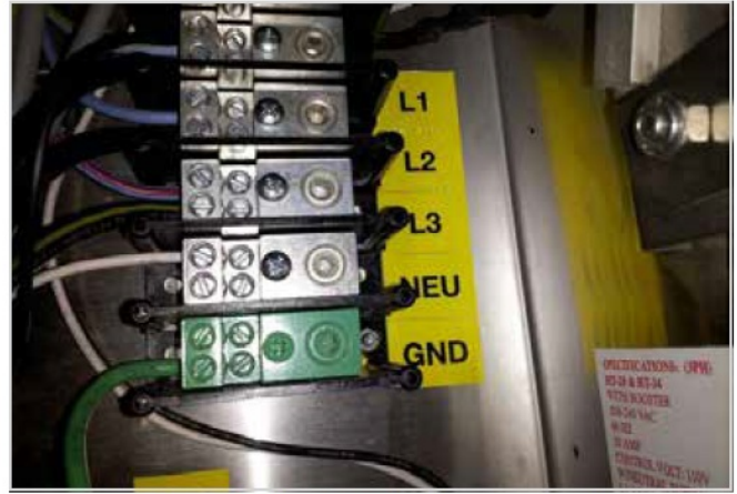
Main distribution block for incoming 5-wire
