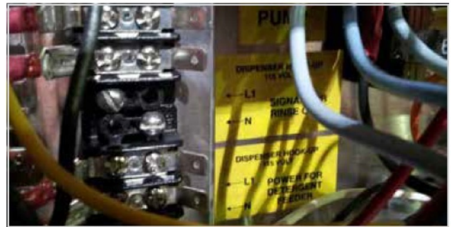
Showing dispenser signal connection terminals
